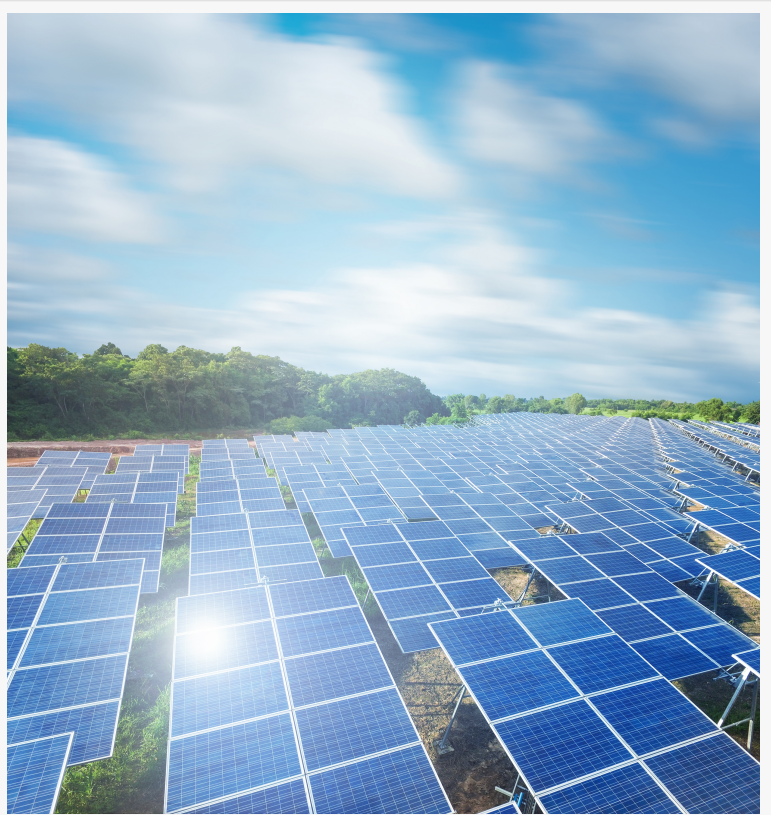
Solar farms like this are driving the future of energy
