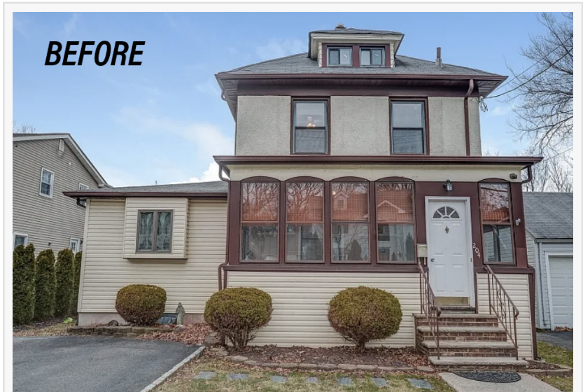
Photo of the house in Cranford before stucco project
