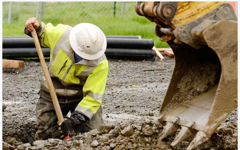
Industry experts estimate that nearly 80% of leak locations found using acoustic sensors are dry holes, i.e. false-positive readings where no leak was found.
