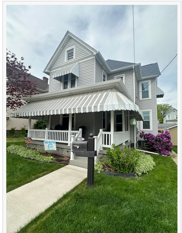
Exterior Painting Perryopolis
