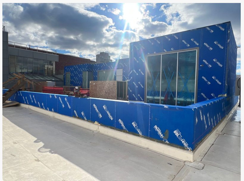
New 5,200 sq ft stucco installation project in Brooklyn, NY
