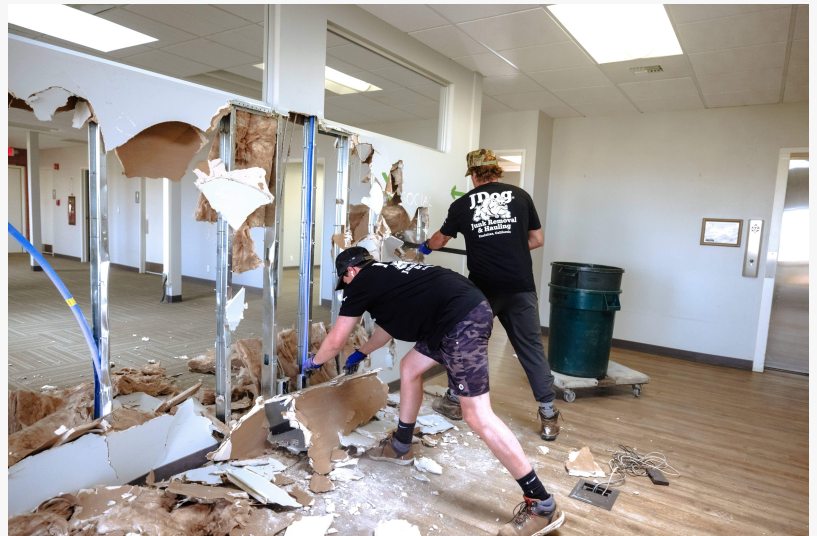
JDog Encinitas Team in Action – Tackling Demolition with Precision
