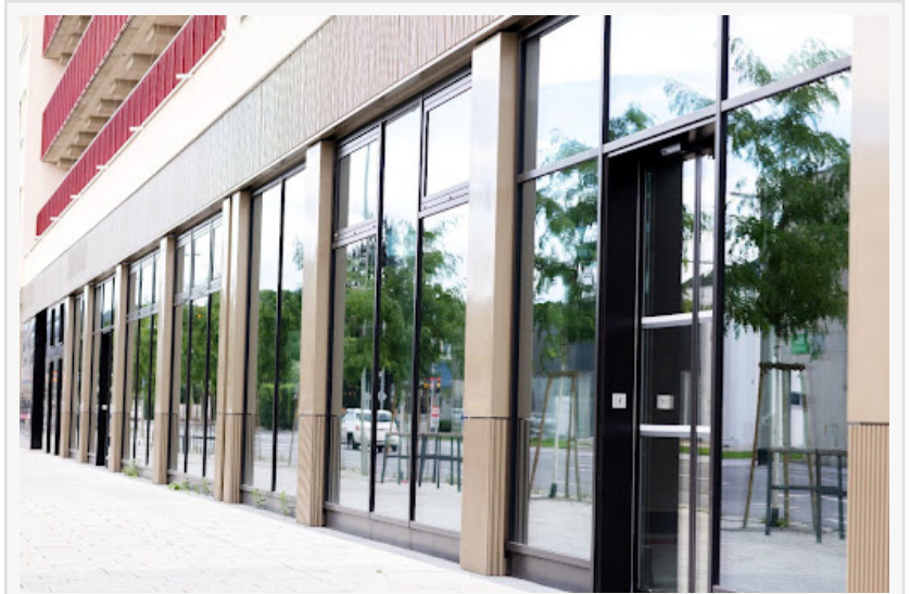
A modern glass facade of a ground-floor commercial building featuring high-quality glass and door installations.
