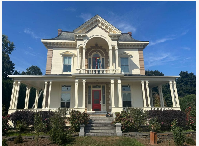
Exterior Painting in Buckland
