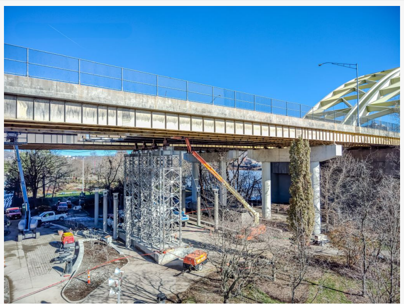
Acrow 700XS Towers on I-471 Ohio
