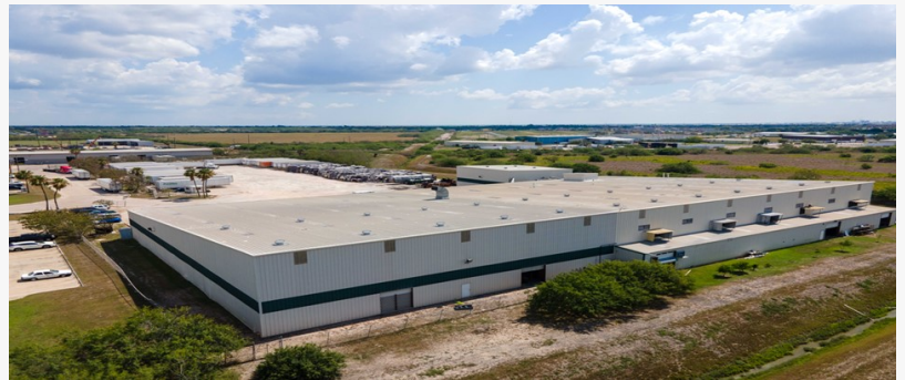
Leigh Fiber facility in Brownsville, Texas Facility
