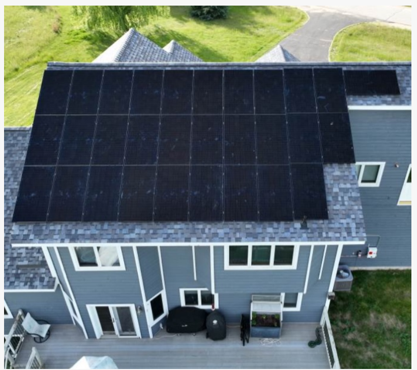
Wolf River Electric - Fully Paneled Roof
