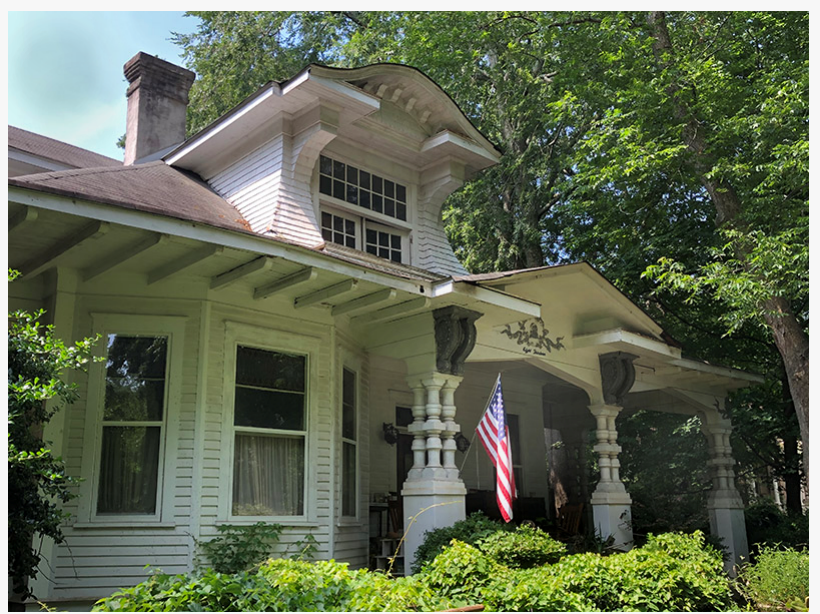
This 130-year Queen Anne home is threatened by a high-voltage transmission line along its side yard.
