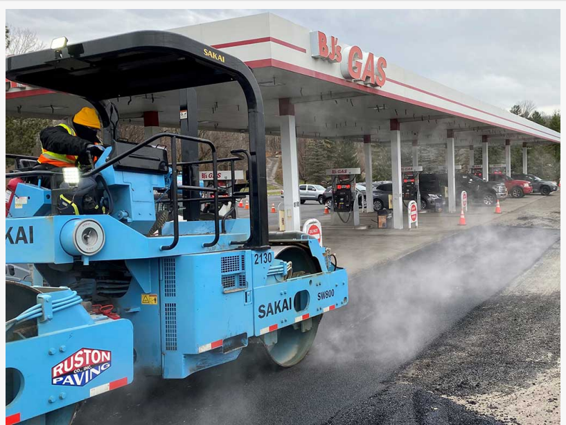
Paving company crews from Ruston Paving rolling new parking lot asphalt
