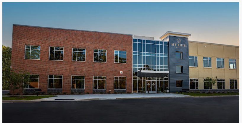
New Waters Recovery Building
