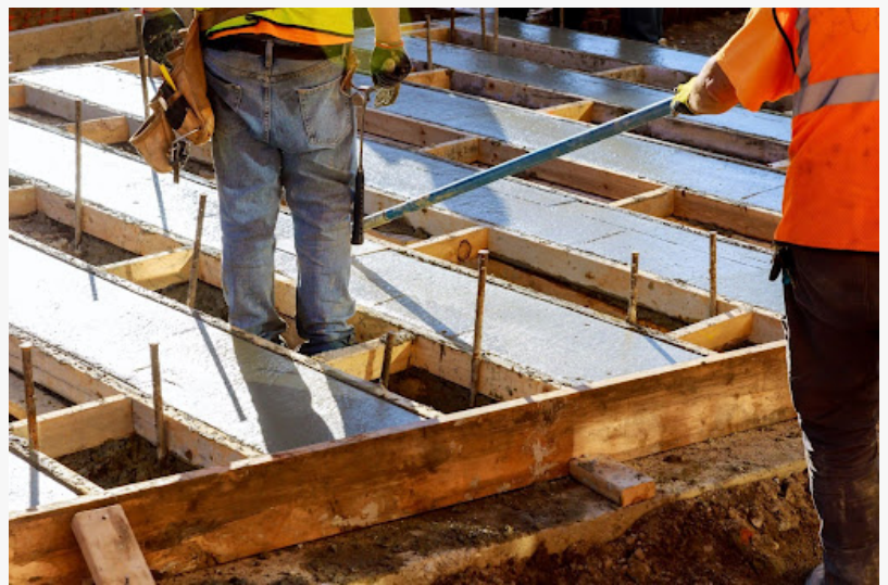
Columbia Concrete Provides Reliable Concrete Foundation Services for South Carolina Customers
