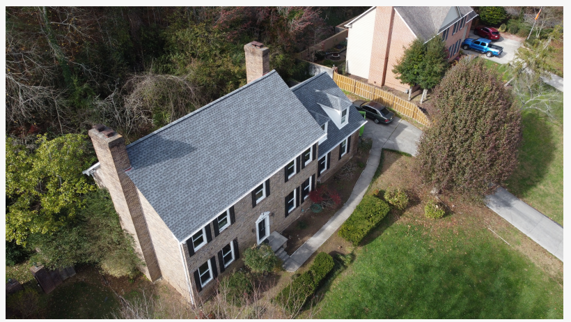
residential roofing client photo
