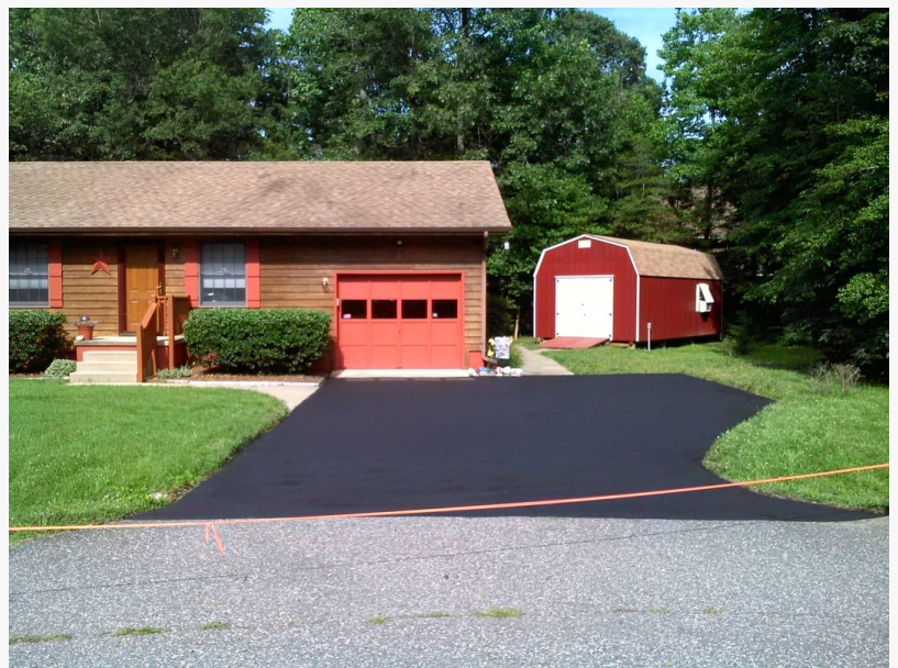
Asphalt Driveway Paving Philadelphia, PA
