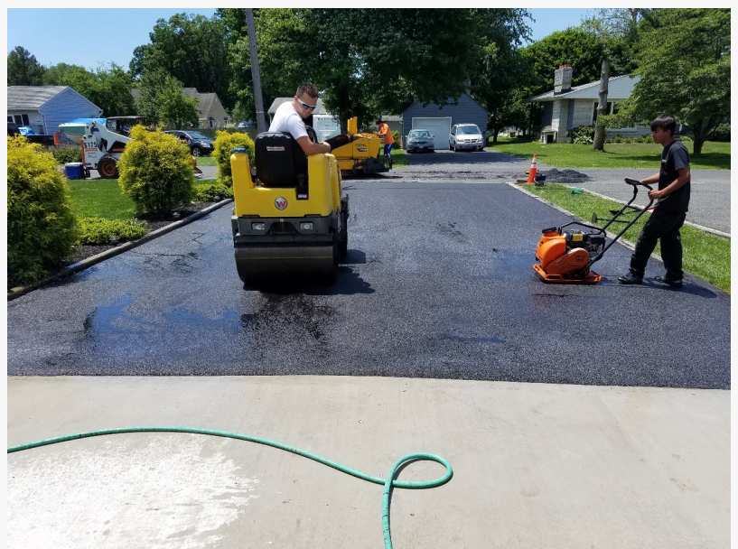
Asphalt Driveway Paving in Glen Mills, PA
