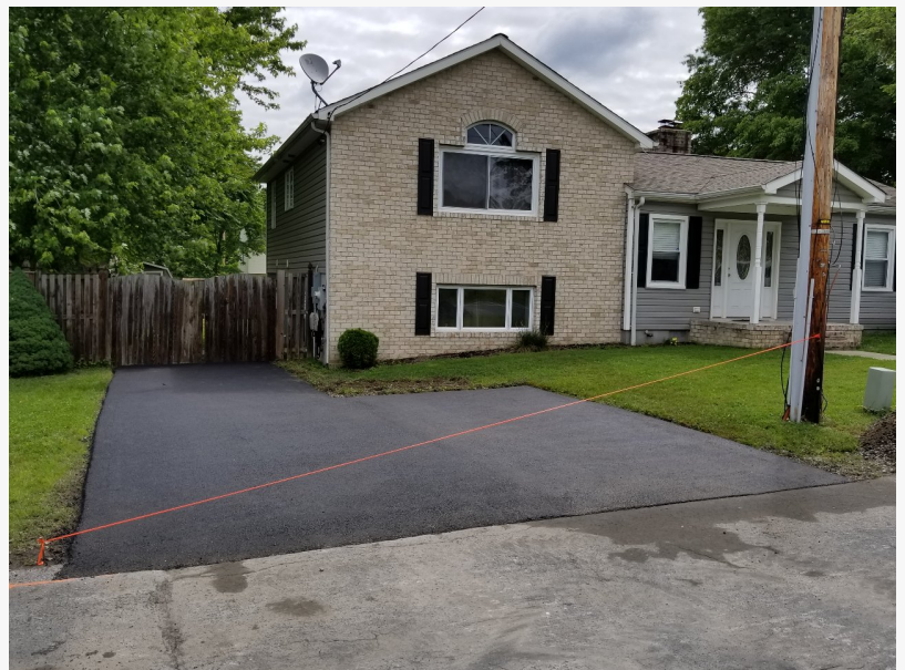
Asphalt Driveway Paving in Cherry Hill, NJ
