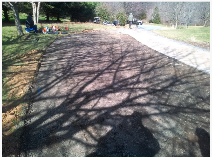
Asphalt Driveway Paving in Elkton, MD
