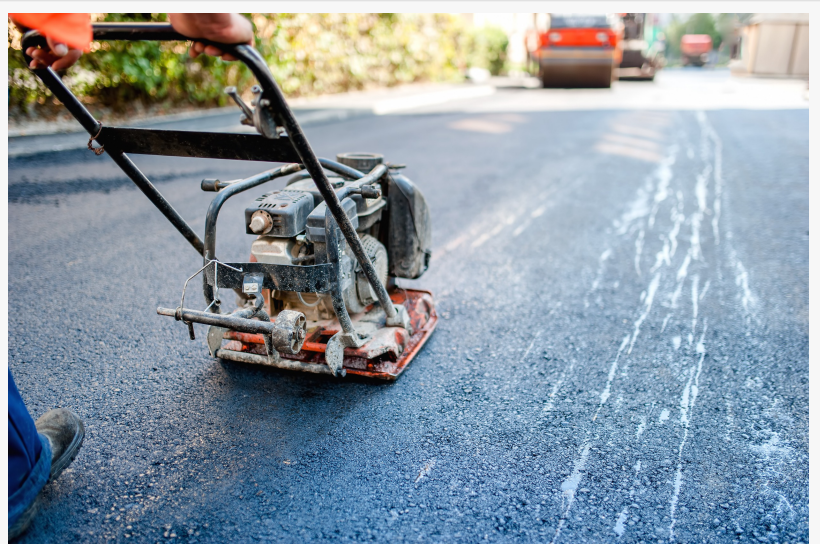
Asphalt Driveway Paving in Coatesville, PA
