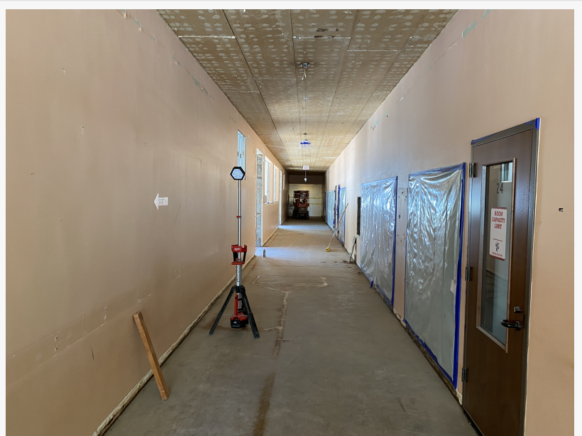
Hallway and Classrooms Renovated from top to bottom
