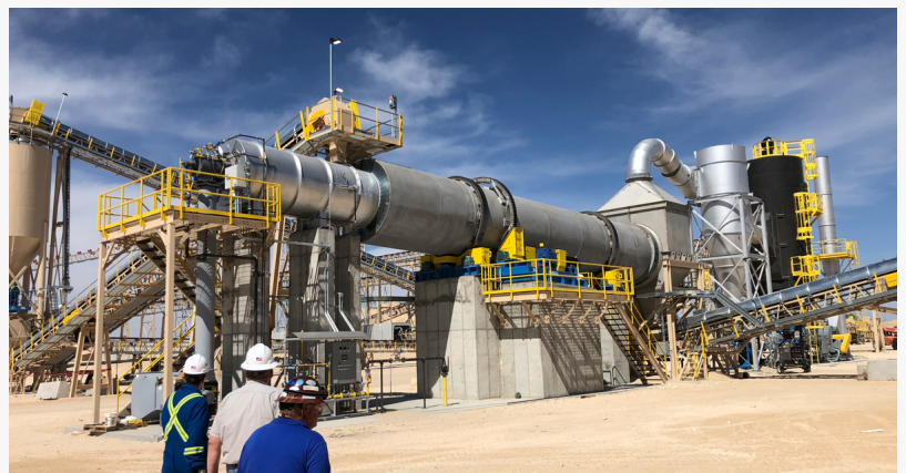
A FECCO Customer Service Engineer begins a walkthrough of a rotary dryer
