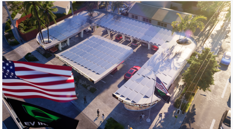
EVII Mission Hills EV Charging Hub
