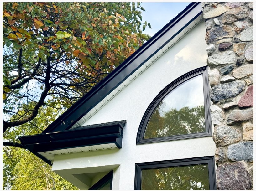
Close-up of the stucco system on the front of the house
