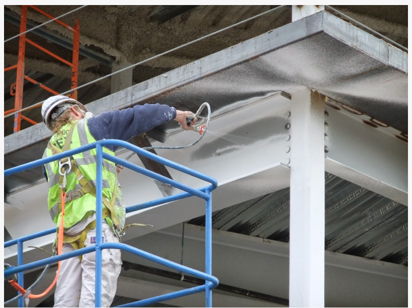
Fire Protection Coating Market
