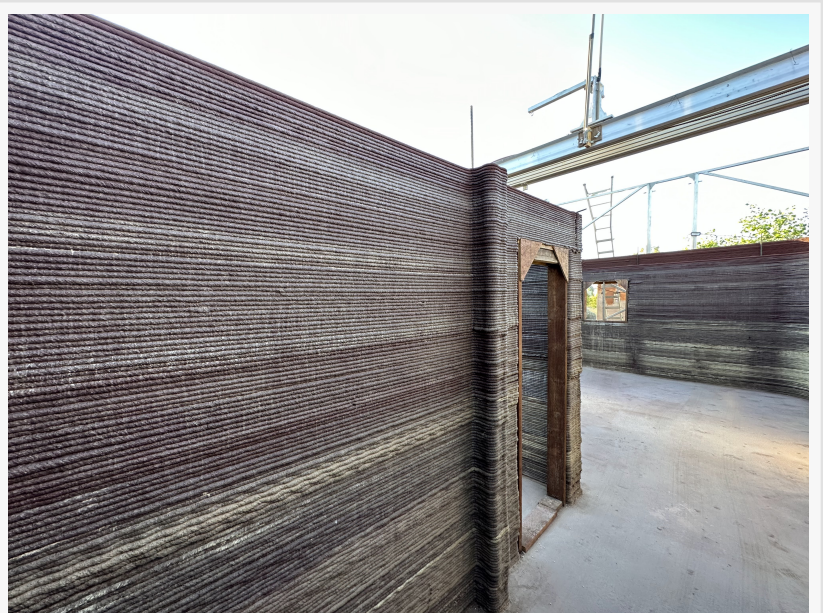
3D-printed walls of a house with RENCA geopolymer cementless mortar.
