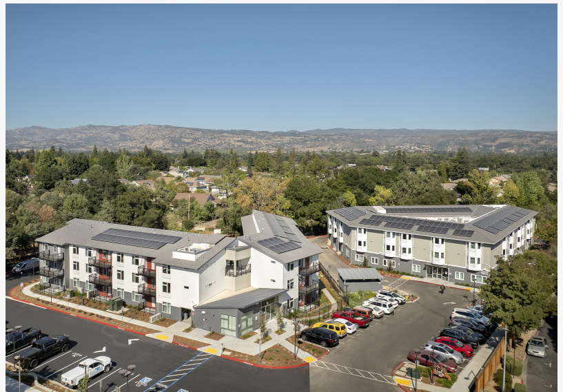
Aerial photo of Heritage House & Valle Verde Apartments
