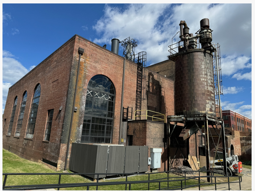
The Power Plant at Liberty
