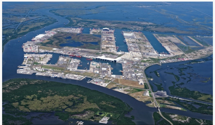
Port Fourchon is a multi-use coastal port that functions primarily as a land base for multiple offshore energy support service companies.
