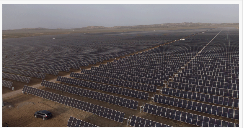
Jicarilla 1 Solar power plant in the Jicarilla Apache Nation in New Mexico.
