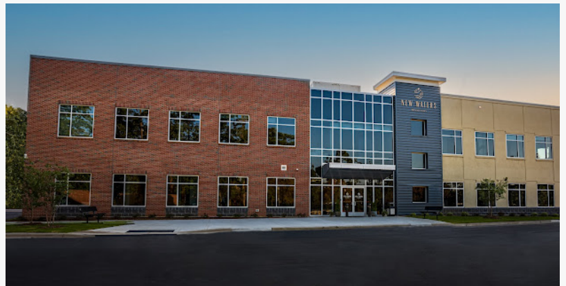
New Waters Recovery Building
