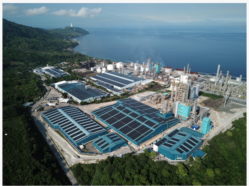
Upgrade Energy Philippines (UGEP) installed the largest rooftop solar for own consumption in the Philippines
