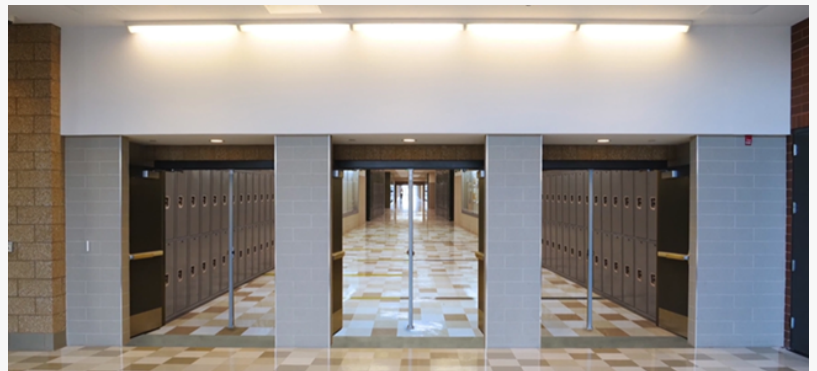
Before: A school hallway lined with closed, traditional-style doors.
