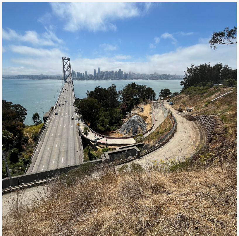
Yerba Buena Island Road Improvement Project
