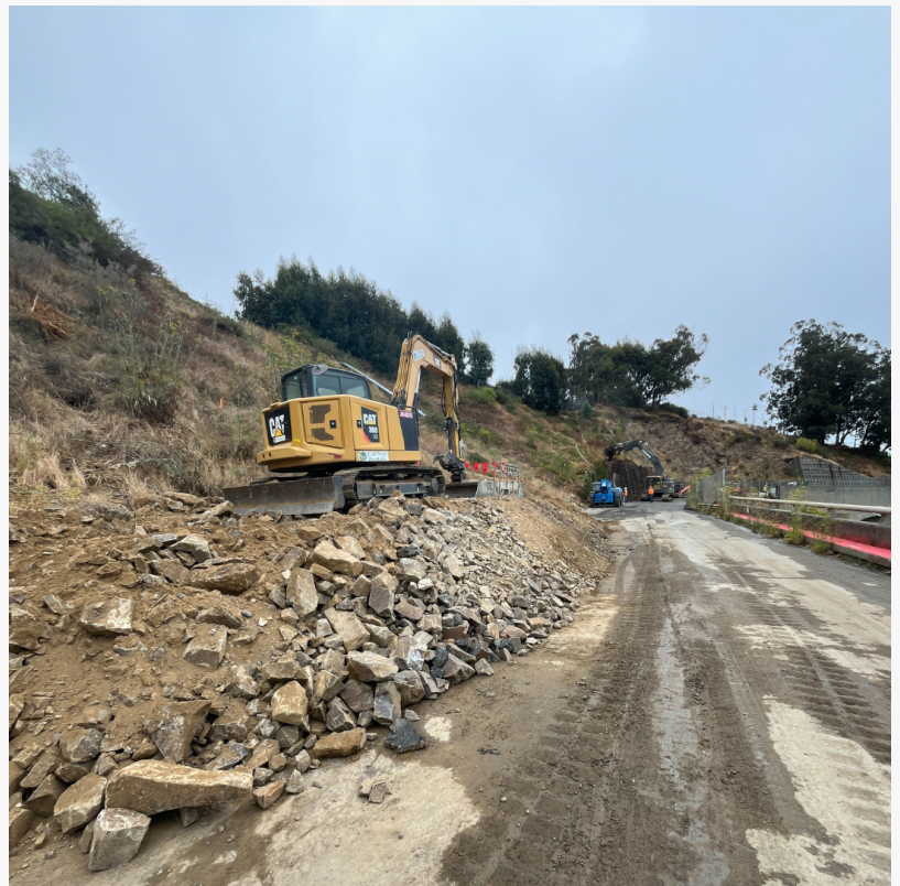
Yerba Buena Soil Grading
