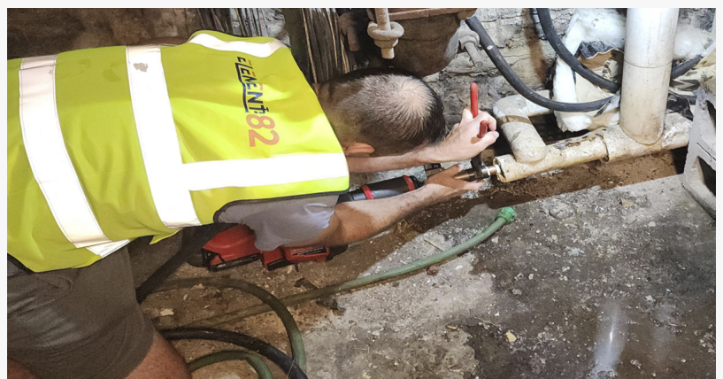
Element 82's President, David Kinsella, performing a SWORDFISH basement entry for an underground water service line assessment.
