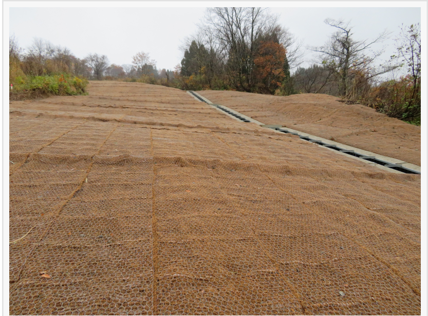
Coir netting used for erosion control solutions
