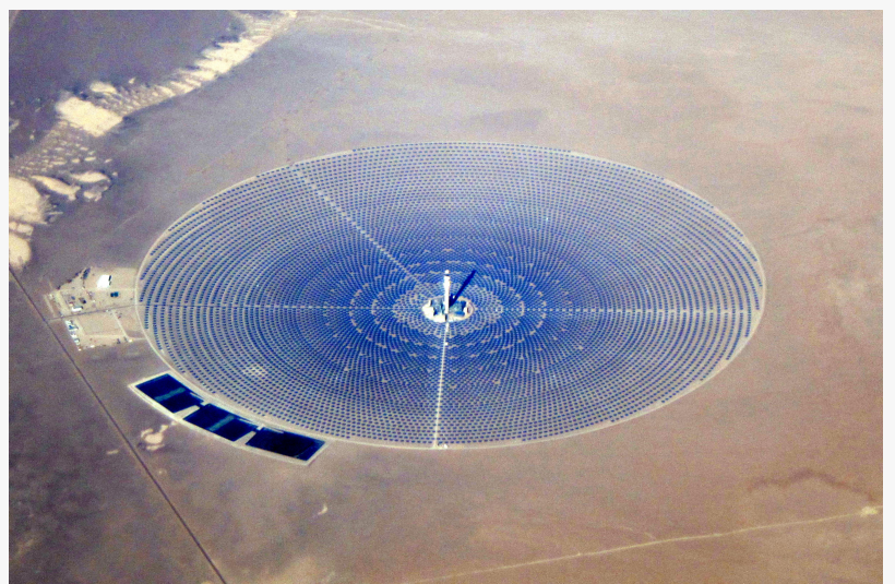
Concentrated Solar Power
