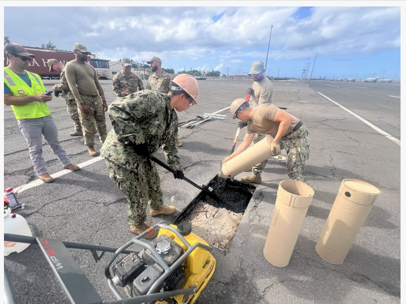
Warfighters using HOTPOD to patch hole
