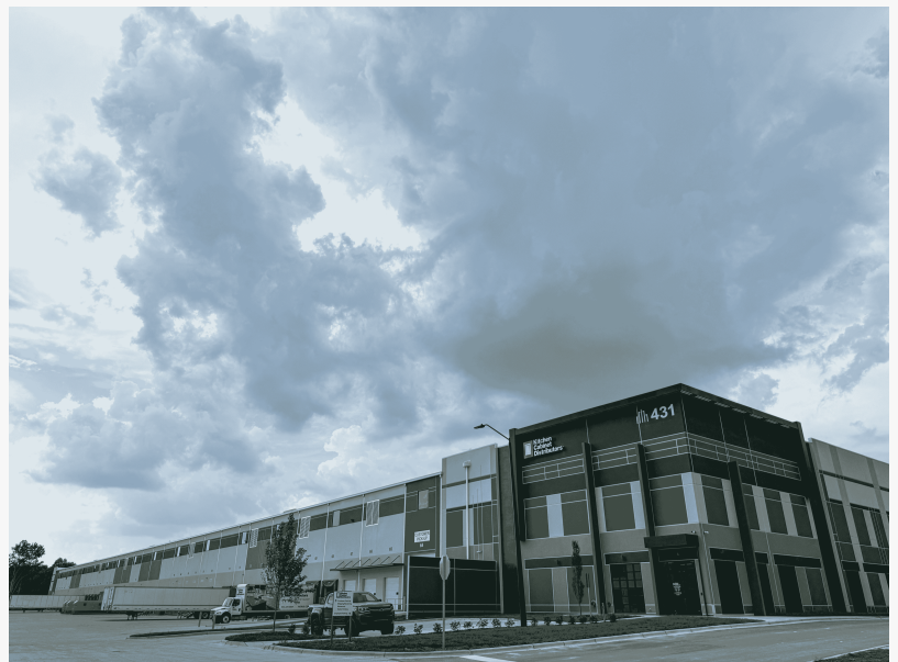
The new Kitchen Cabinet Distributors headquarters. Located in Raleigh, NC.
