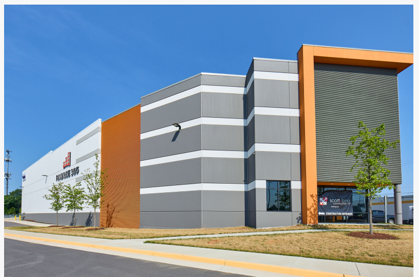
Scott-Long Construction Completes Relocation Project For Largest Fire Protection Supplier
