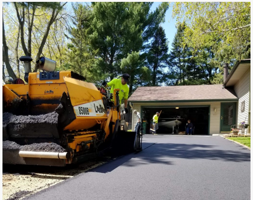
Asphalt Driveway Paving in Arlington, VA
