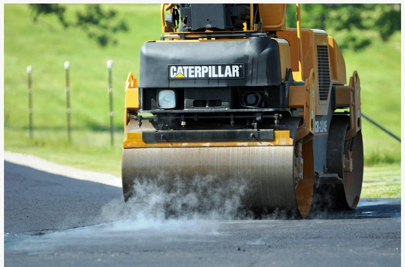
Asphalt Driveway Paving in Alexandria, VA
