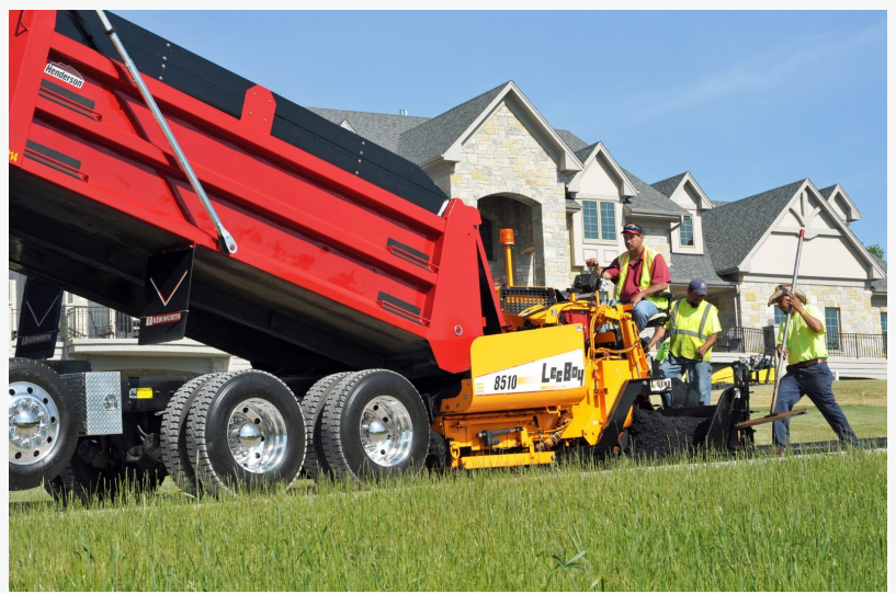
Asphalt Driveway Paving in Fairfax, VA
