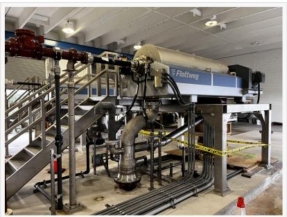
Numerous centrifuges are used worldwide in a wide variety of wastewater treatment applications in sewage treatment plants.
