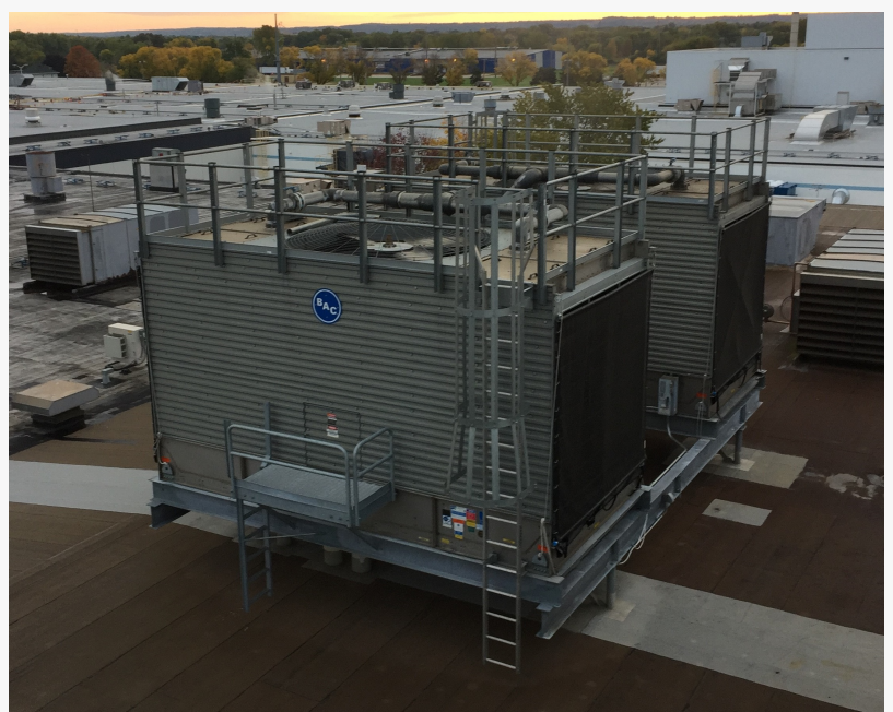
Industrial Cooling Towers Being Installed
