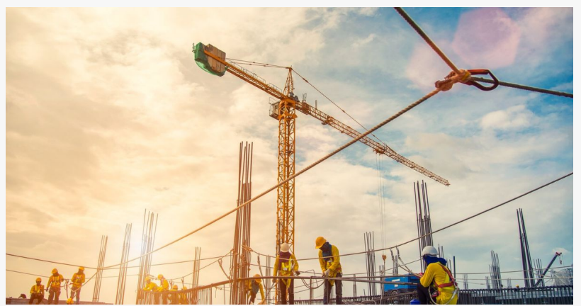
On-Going Construction Site
