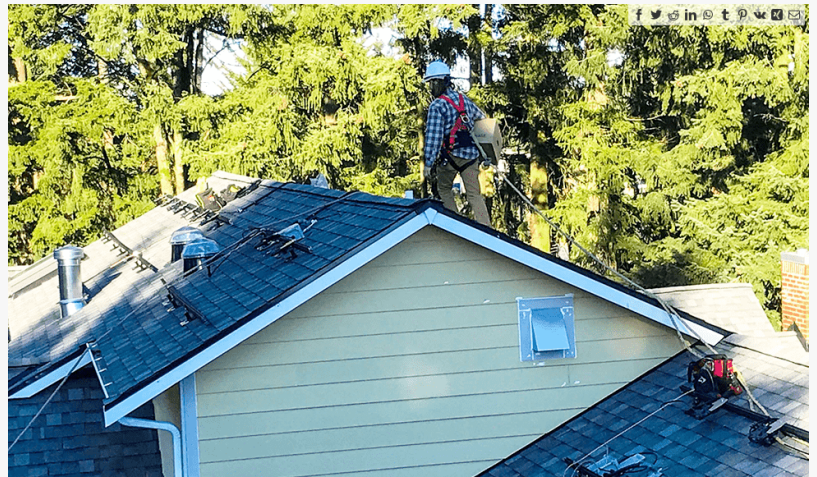
Sunergy Systems Installing Solar
