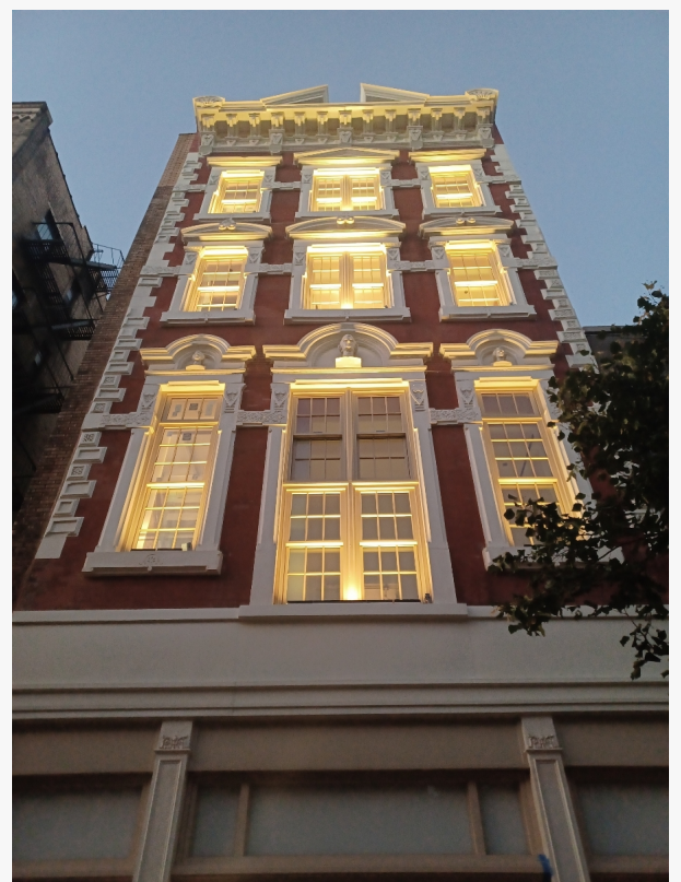
Gotham Metal Works helped to preserve the historic façade of the landmark building at 74A East 4th Street.
