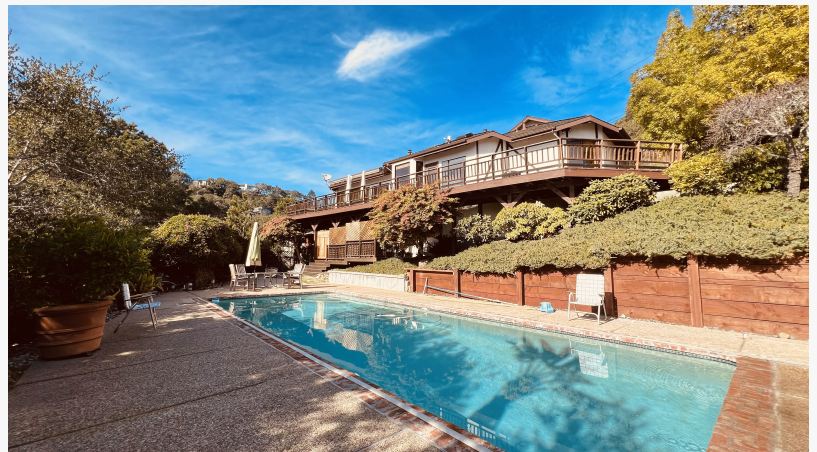
Wi-Fi Testhouse villa for wireless technology
