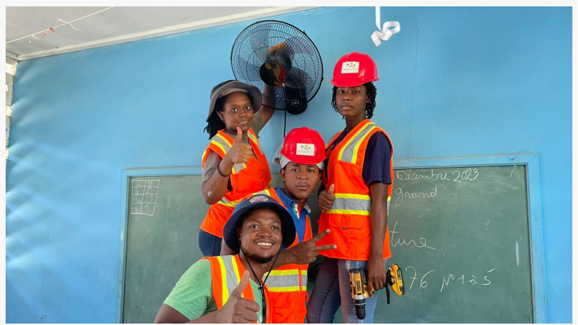
Rural Haitian School gets fans installed along with solar energy
