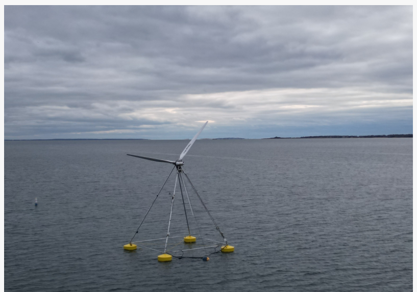
Floating offshore wind turbine prototype, produced by T-Omega Wind
