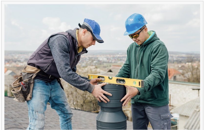
Two men working on chimney repairs.
