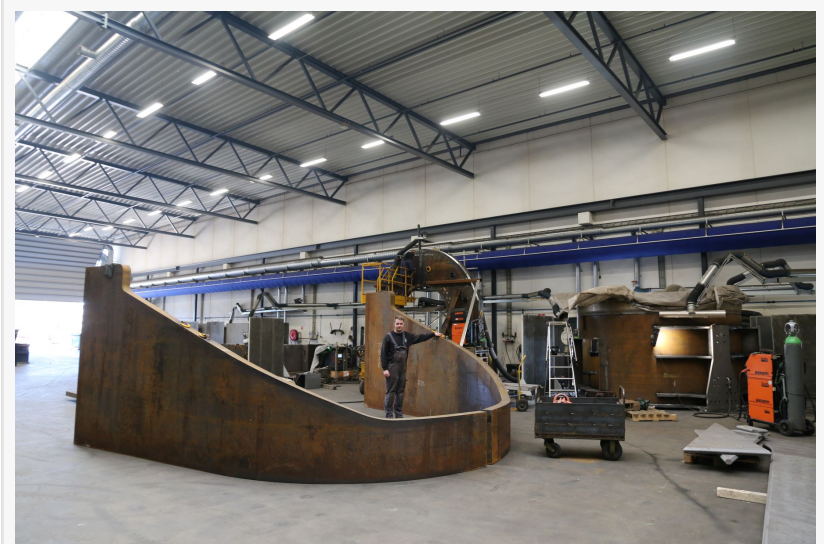
The first steel structure for R&D Test Systems' new end-of-line test rig has been made.
