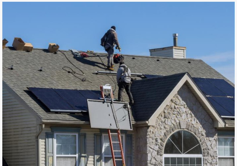
Roof repair for a local Pawtucket homeowner
