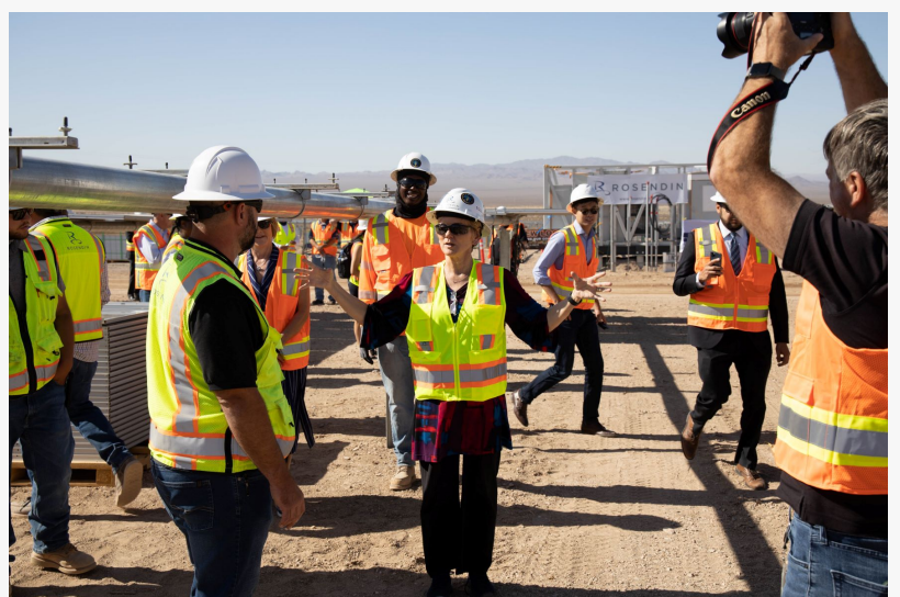
Energy Secretary Jennifer Granholm tours Townsite Solar and Storage in Nevada
